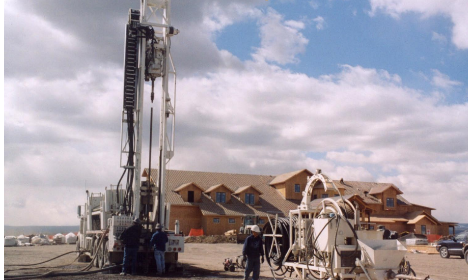
Project Site with Drilling Rigs
